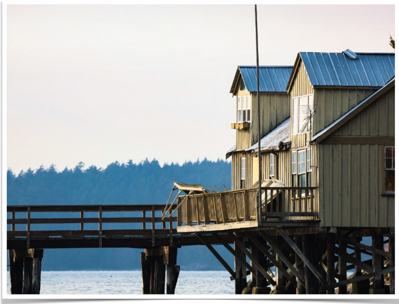
"The Shed" at Port Washington
